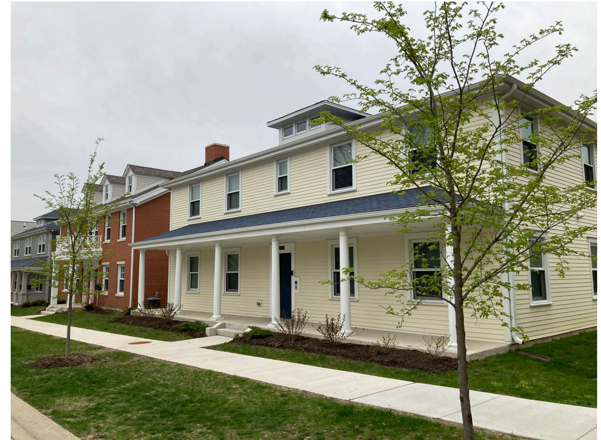
1212 Larkin Apartments, Elgin Developer: Full Circle Communities
